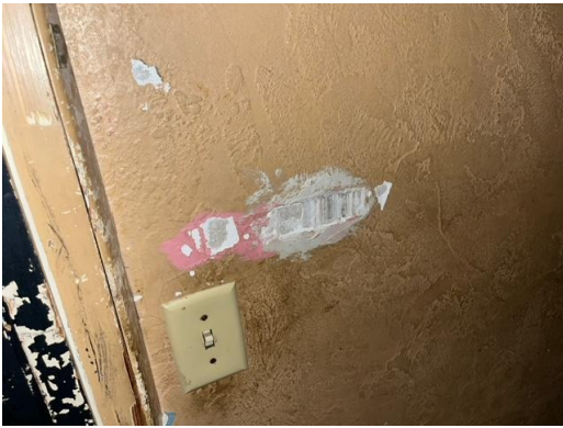
514-3 Plaster/Rough Coat Typical Interior Walls/Ceilings
