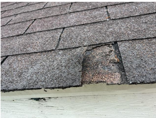
514-5 Asphalt Shingle Typical Exterior Roof
